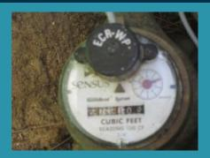
Photo caption: This is a sample of one of the old analog water meters being replaced by a new digital version
