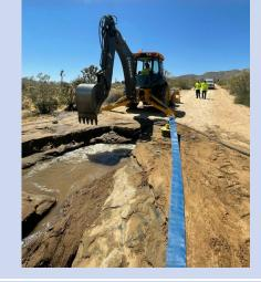
our call center at 9:30AM. With the help of our three trucks, a tractor and a dump truck, a water vacuum system and a water pump on site with five employees, the massive leak was repaired at approximately 6:30PM.
