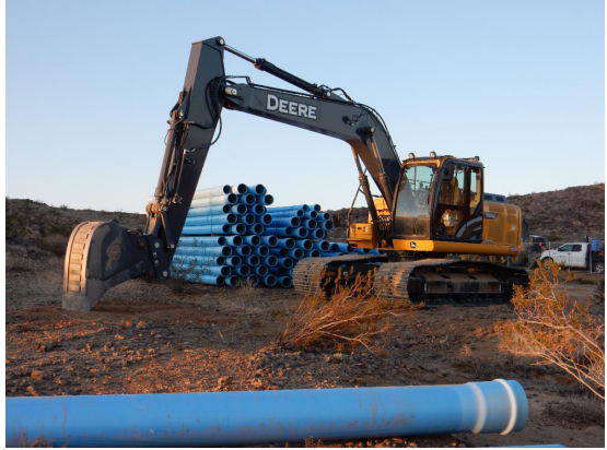
Photo: Installing new pipeline on the Tilford Project: Phase One.
