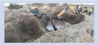
**Photo Caption:** All crews responded to a major water feed-line break at Well 14 that was located 30 feet deep! The repairs began at 9AM on August 6, and concluded at 4AM on August 7. Controlled shut-downs interrupted water service to a few customers, and impacted water pressure to many others.
