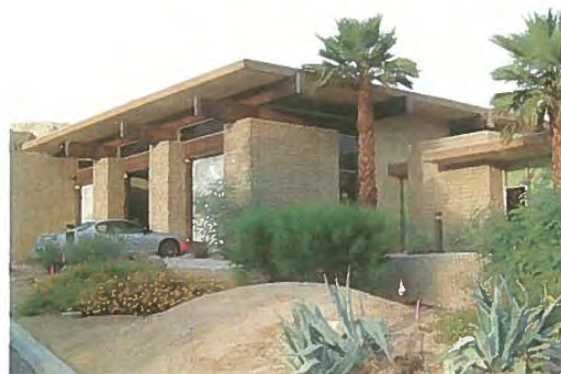
FIRE STATION 50 Renovation, Rancho Mirage, California
