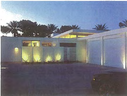
Zoll Residence. Motorcourt & Glass Screen
